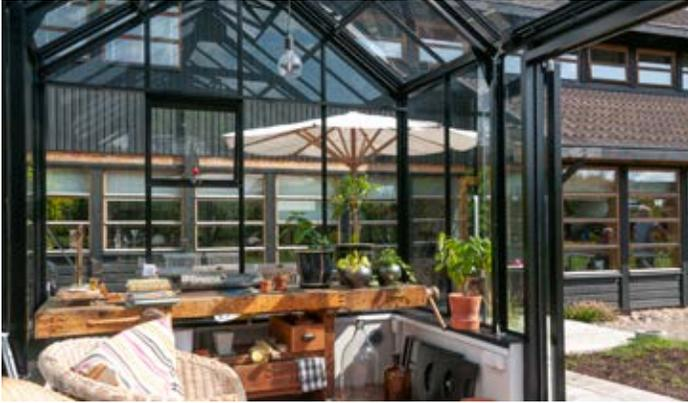
**6MM Full Sheet Glass:** One solid sheet of tempered safety glass in every greenhouse bay which is double the thickness of our standard 3mm Single Glass. Offering similar light transmission benefits comparable to standard 3mm, the 6mm option also adds additional strength. 6mm Full Sheet Glass also provides you with a beautifully seamless look that will elevate your greenhouse's appearance.
