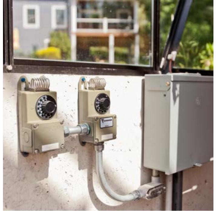
Planning on using an electric heater or grow lights in your greenhouse? Colder climates and larger greenhouses may need a 220-volt heater in winter. This heater requires more voltage than a standard circuit provides. Connect with your electrician to see if you need additional power.
