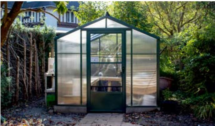
**A Cool House:** If you live in a mild climate and want to winter over your plants, a cool house is probably your perfect fit. A greenhouse with single glass sidewalls and a twinwall polycarbonate roof allows for optimal growth in the spring and summer. This greenhouse would maintain a night temperature of 40 - 45 Fahrenheit (5 - 7 Celsius).
